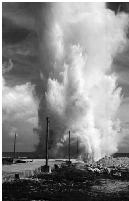
Figure 34.1 Shallow underwater blast undertaken for reef passage clearance using a slowly detonating explosive (ammonium nitrate – fuel oil mixture). Note the large plume.
