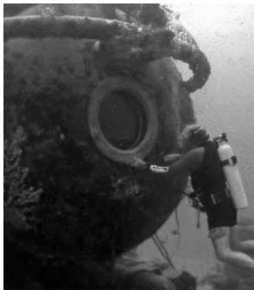
Figure 67.1 A diver working to maintain the outside of Aquarius by cleaning off marine growth. He is using a hookah rig that includes a typical second stage regulator attached to an air hose that leads to Aquarius and an air storage tank. A secondary 'bail-out' bottle is on his back for safety if problems develop with the hookah rig. (From National Oceanic and Atmospheric Administration. http://oceanexplorer.noaa.gov/technology/diving/aquarius/aquarius.html .)
